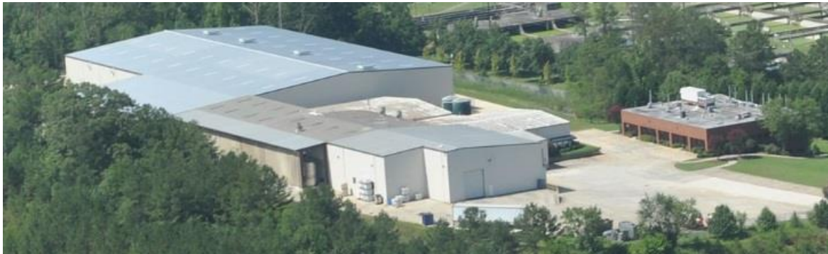
Walnut Grove Site – Cartersville, GA
